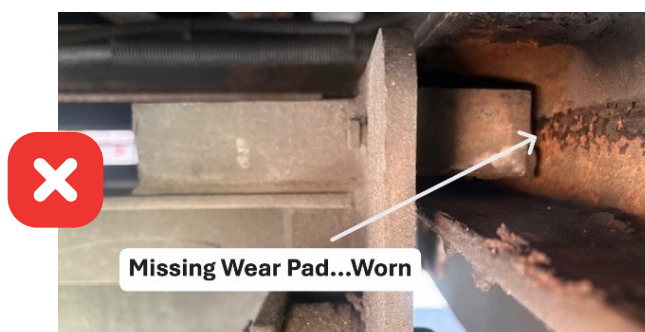
Bad Skid Wear Pad Adjustment
