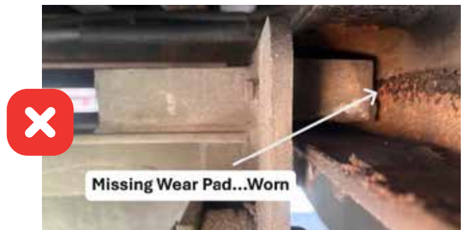
Bad Skid Wear Pad Adjustment
